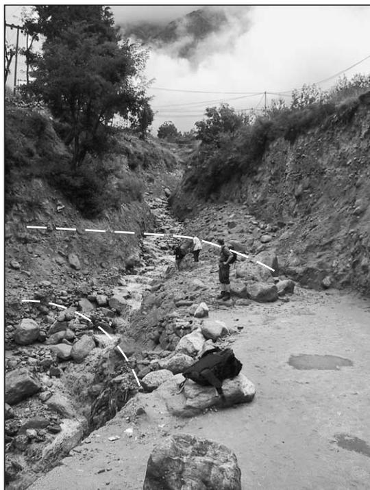
Fig. 6. Remnants of a debris-flow in the village of Sangla, Baspa Valley during the 2002 AMY (31.8.2002). White dashed lines indicate location of destroyed road. Note levee material related to debris flow showing the thickness of the flow.
